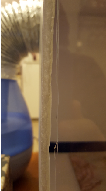
Figure 36: Walls are starting to warp outward.
